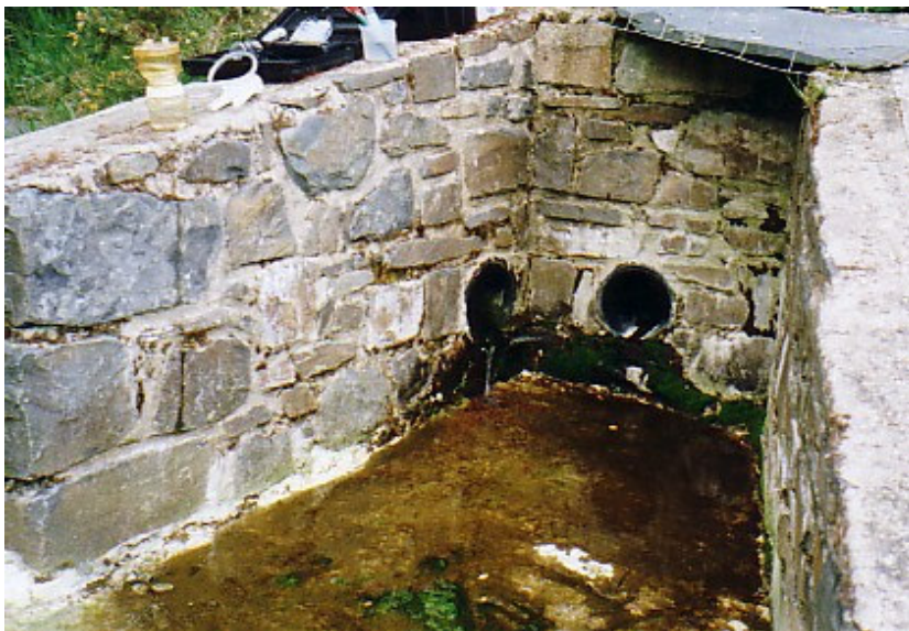
Figure 2.9. Outlet pipes at Bwlch.
