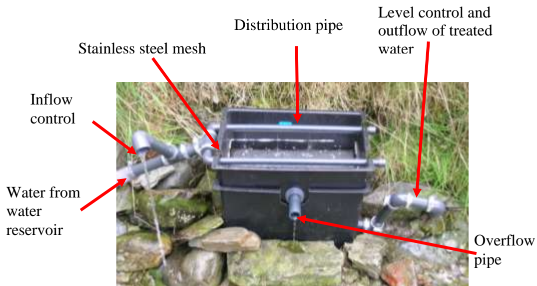
Figure 7.2. 1 L/minute treatment plant at Bwlch.
